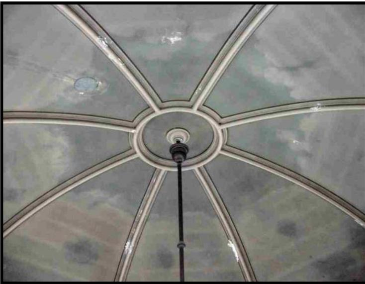
*Above: Looking up at the dome. It is easy to see the discoloration. The spots of bright white in each picture are areas where the plaster has fallen.*
