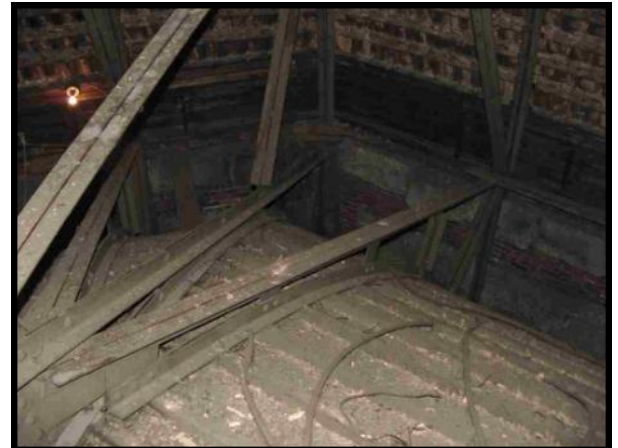
Left & Right: A view inside the dome. This is an open area that is between the interior and exterior. This open area houses the wench system that raises and lowers the large chandelier to allow for cleaning and replacement of light bulbs. As part of the repair and restoration this area will be professionally cleaned by the paint conservator.
