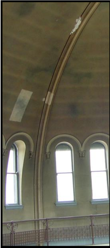
Left: The two square bright spots are an indication of how badly the paint has become stained over the years. This area was cleaned 3 years ago as a test to reveal the true color of the paint.
