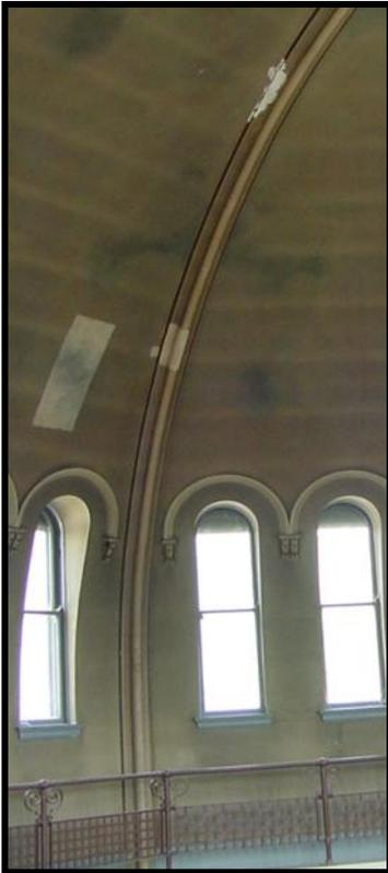
of the paint. This is caused by moisture that migrates through the paint from the back side carrying dirt with it. Over many years this, along with smoking that was allowed at the courthouse, has caused the dome to become severely discolored.
