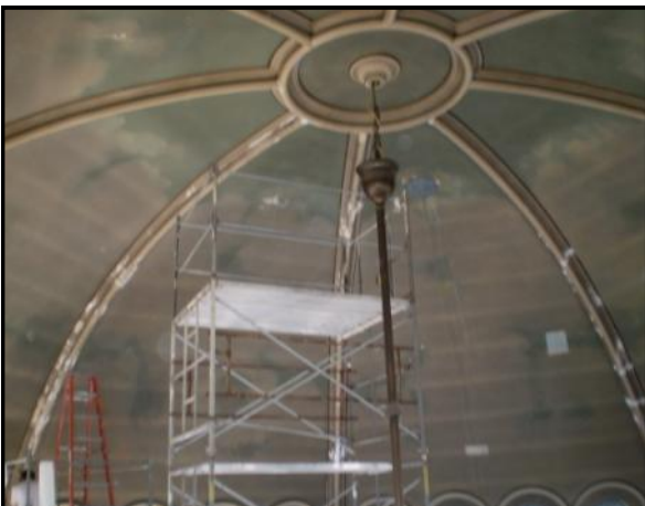
Left: Scaffolding in place to repair the plaster.
