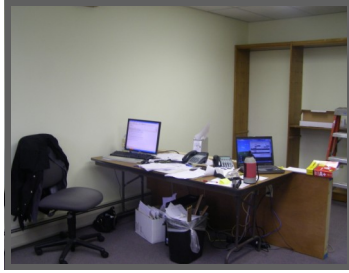
Above: Work continues on the I.T. office
