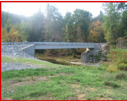
Bradford County Bridge #32 North Towanda Township
